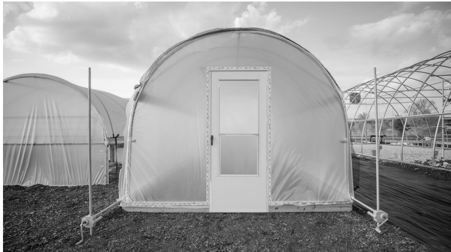
Fig. 6 End Wall With Door Frame and Door
